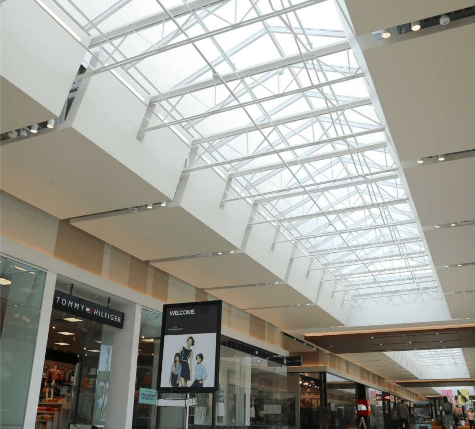
Image: Over 250' of Gable Ridge custom skylights at the Ontario Mills Mall in Ontario, CA. Contractor: Moorefield Construction
