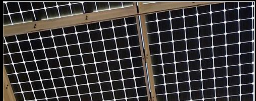
Smaller spacing of solar cells, less day lighting, more sun control, higher efficiency per SqFt.
