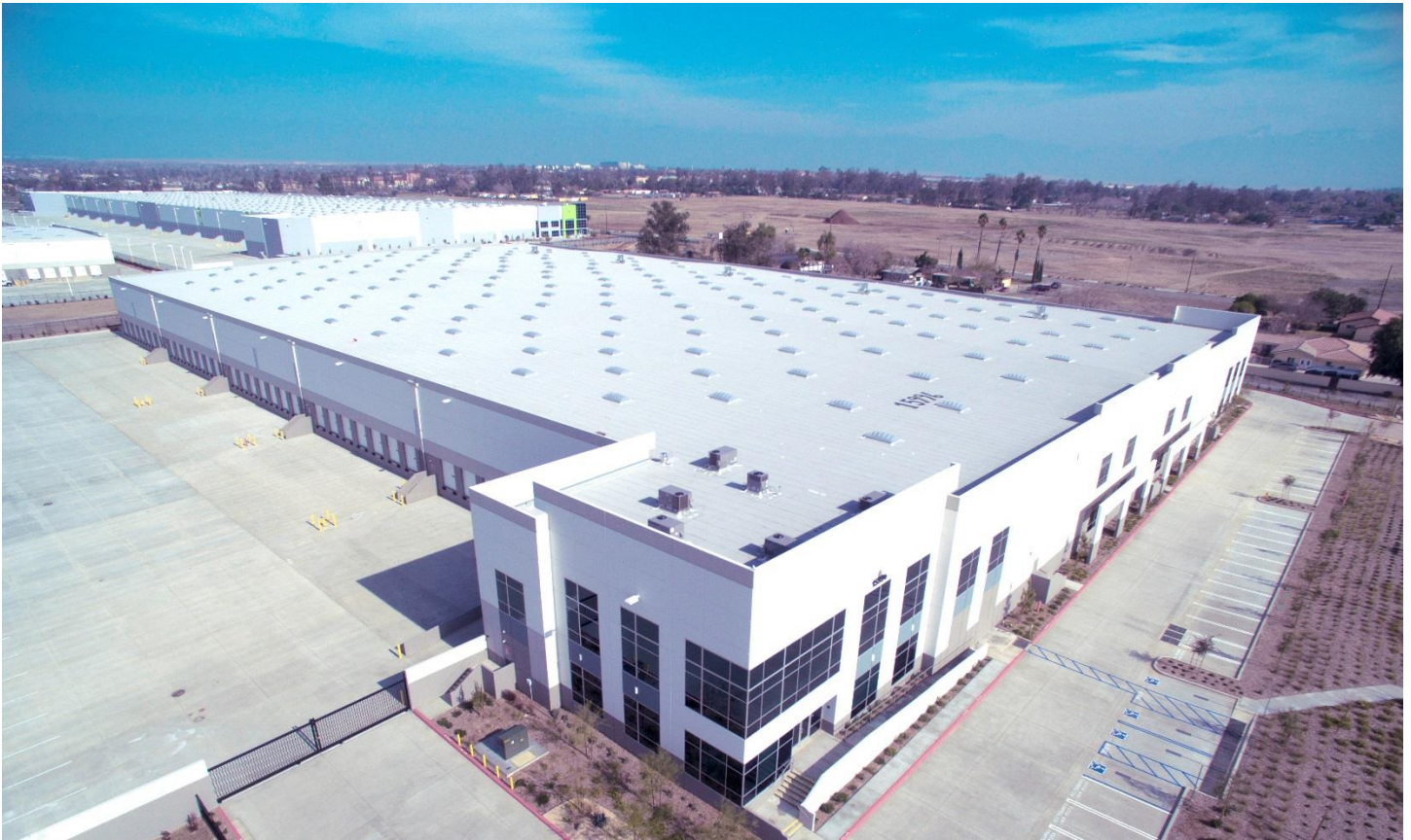
150 SKYRPO Illuminator Unit Skylights, ICC-ES (ESR-3837) provide ample daylighting for this logistics facility in Fontana, CA.
