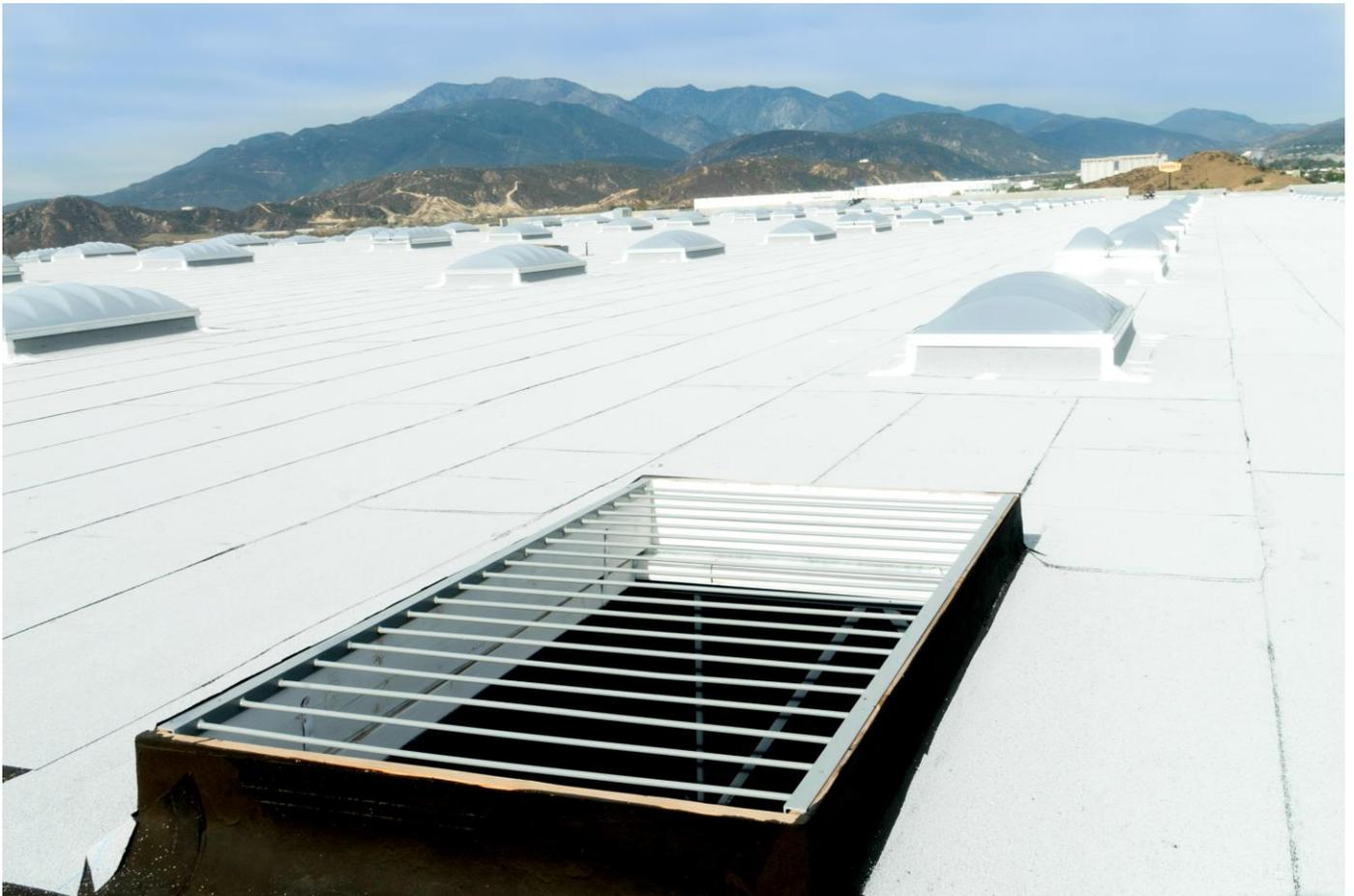
Security bars sit underneath the skylights and provide fall protection and security for building owners and occupants.
